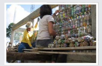
"Eco-bricks" are plastic bottles densely packed with inorganic trash (for example, plastic bags, chip packets, and polystyrene). Community members gather the trash and stuffs the eco-bricks to begin the construction process. Masons then sandwich the eco-bricks between chicken wire and cover them with cement to form the walls of the new bottle school.
